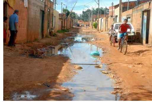
An open sewer in a Brazilian favela.
